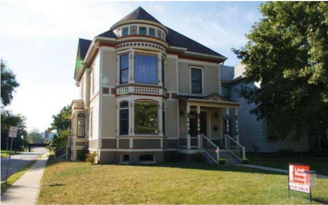
This fully restored home at 901 N. Fifth St., now on the market for sale, is one of the “after” houses featured on Enos Park’s Oct. 5 “Before and After House Tour.” PHOTO BY JOE COPLEY
