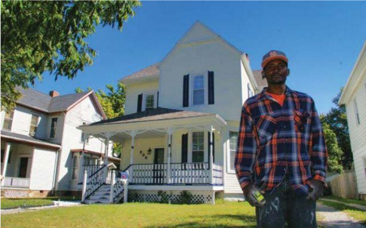
Before Jermaine Ward bought this house on North Fifth from Enos Park Development it had been considered a candidate for demolition. But over the past two years Ward, a building contractor, has lovingly restored it as his residence.
